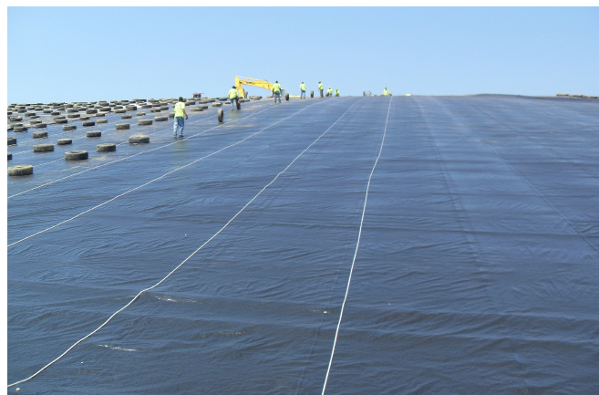
Temporary Rain Shed Cover
