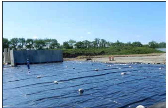
Brownfield Containment Liner
