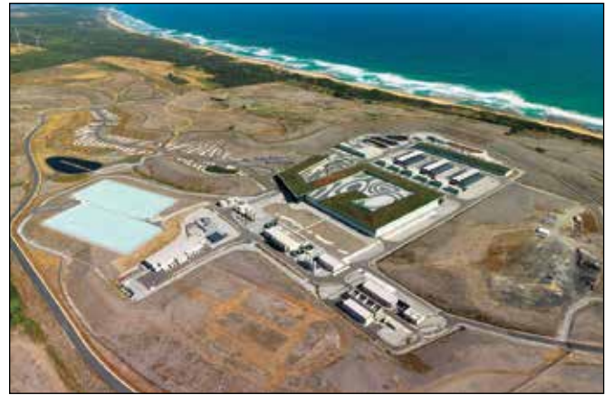
Desalination Plant Cell Liner & Floating Cover
