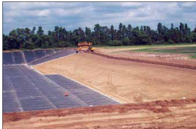
Reservoir Containment Liner
