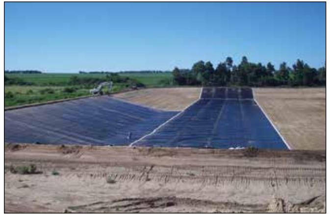
Waste Lagoon Liner
