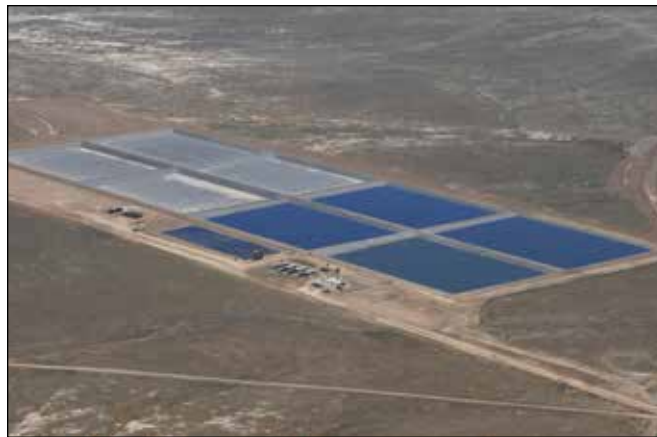
Evaporation Pond Liner
