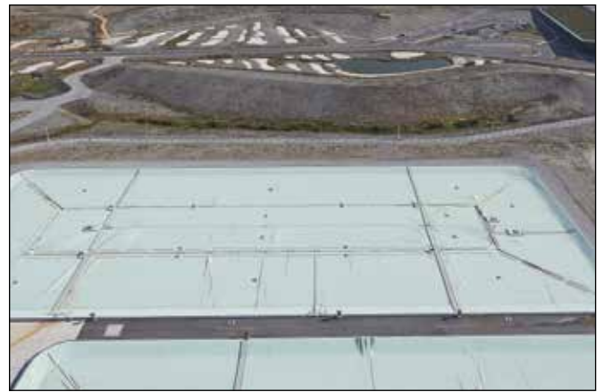
Desalination Plant Cell Liner & Floating Cover
