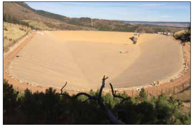
Potable Water Storage Reservoir
