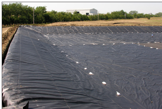
Waste Containment Liner
