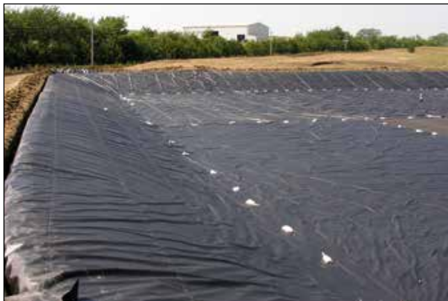
Waste Containment Liner
