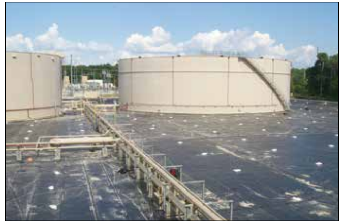
Tank Farm Secondary Containment
