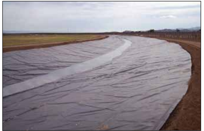
Irrigation Canal Liner
