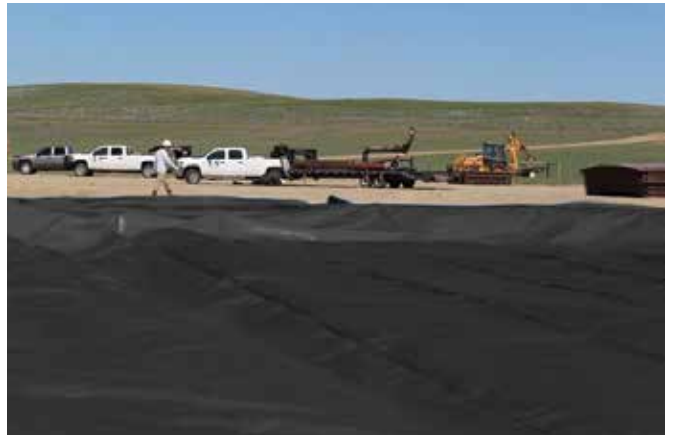
Rig-Site Pad Liner
