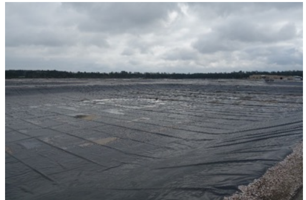
The East Texas Fish Hatchery facility
