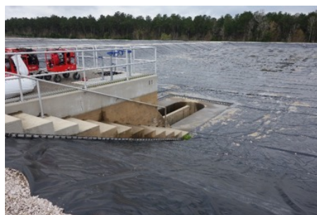
A repaired kettle with the custom-fabricated Rufco 4000B
