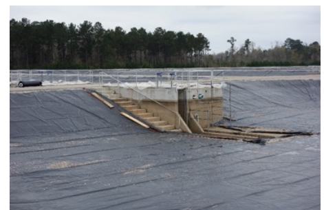
A pond kettle structure with the attachment hardware
