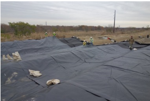
Folded panel of DuraSkrim® K45BT2 being aligned for welding preparation.
