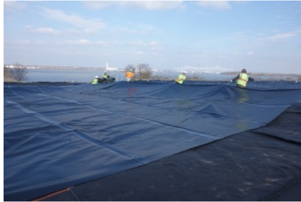
Folded panel of DuraSkrim® K45BT2 being opened for installation.
