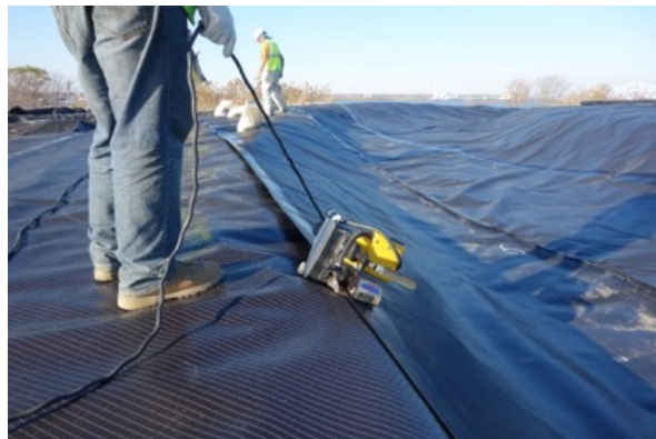
Panel of DuraSkrim® K45BT2 being welded to adjacent panel.
