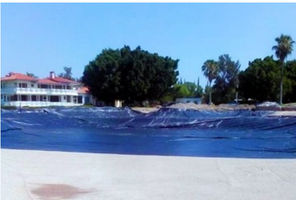
Rapid large fabricated panel deployment.
