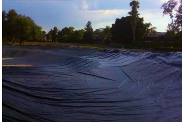
Minimal seam welds to join large panels.
