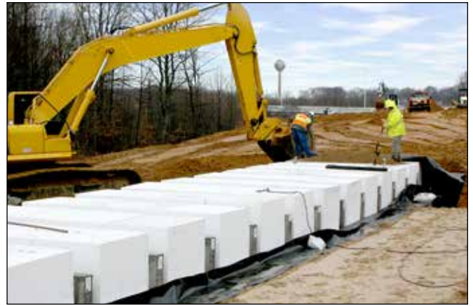
EPS Geofoam Protection
