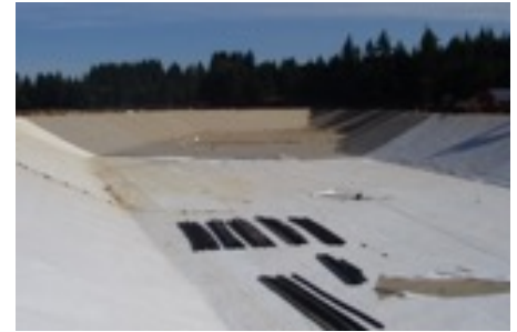
Liner installation – white section
