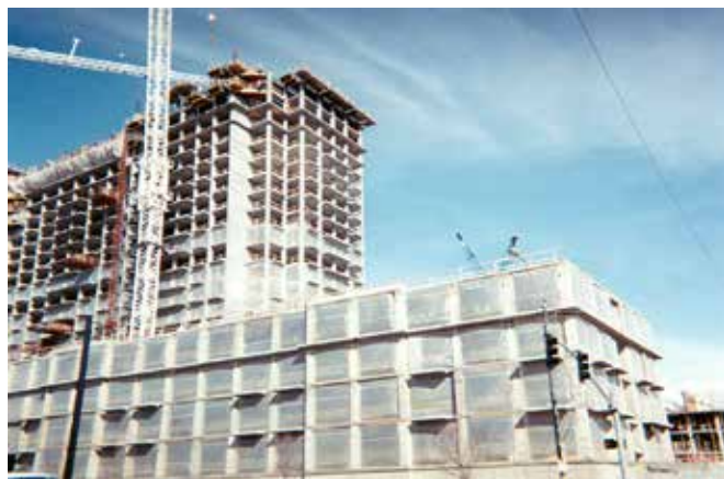
Building Abatement Enclosure
